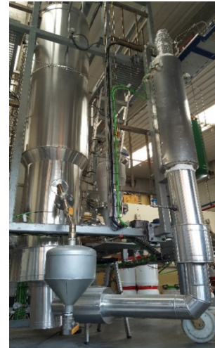
Figure 2. Picture of the BFB gasifier at ICB-CSIC.
