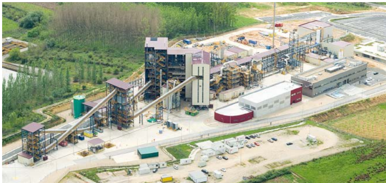
Figure 1. Aerial view of CIUDEN's Technology Development Centre for CO 2 Capture
